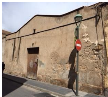
Naus industrials abandonades al carrer Smith.
